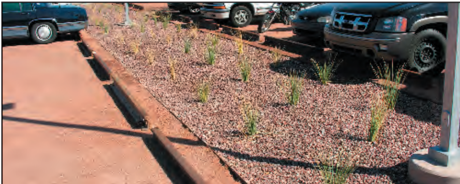
Permeable pavements can reduce stormwater runoff from parking lots.
