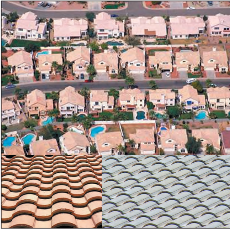
Figure 2-15. Concrete-tiled roofs in the Valley of the Sun. Photos courtesy of National Center of Excellence, Arizona State University.
