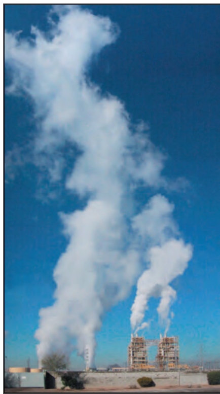
Figure 1-28. Steam cloud generated from cooling towers at APS's Ocotillo thermoelectric power plant in Tempe, AZ (Source: City of Tempe).
