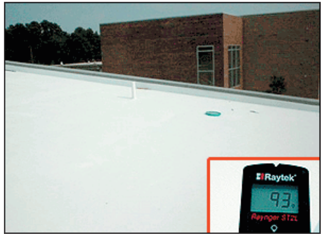
Figure 2-30. Cool roofing on a commercial low sloped roof. The surface temperature was reduced by 85°F after the roof was treated with a liquid applied cool roofing product. Images courtesy of Hydro-Stop, Inc.
