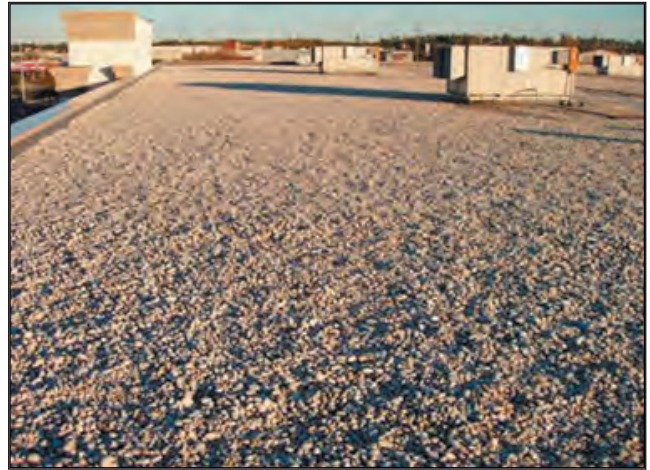
Figure 2-20. Image of a ballasted, loose EPDM roof. Source: NRCA
