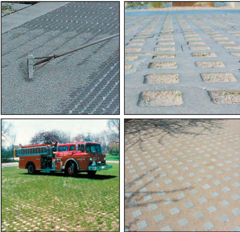
Figure 2-68. Open grid pavements come in a variety of designs and provide a cooler alternative for parking lots and other hardscapes.
