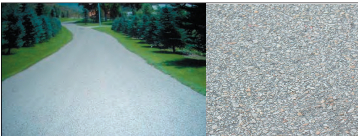
Figure 2-63. A road made of asphalt concrete with reflective aggregates. Courtesy of the Asphalt Pavement Alliance.
