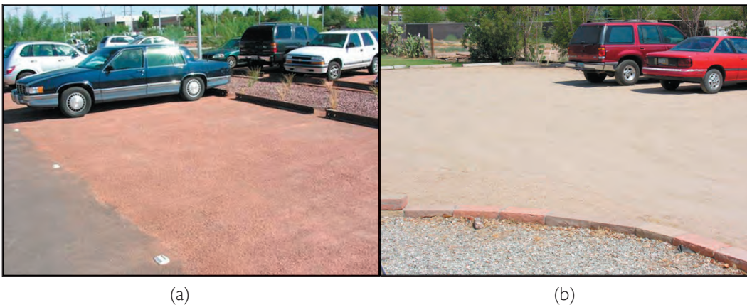
Figure 2-69. Examples of an open grid parking areas comprised of stabilized granite: (a) East Valley Transit Facility, and (b) a residential complex in Tempe, Arizona. Photos courtesy of National Center of Excellence, Arizona State University.
