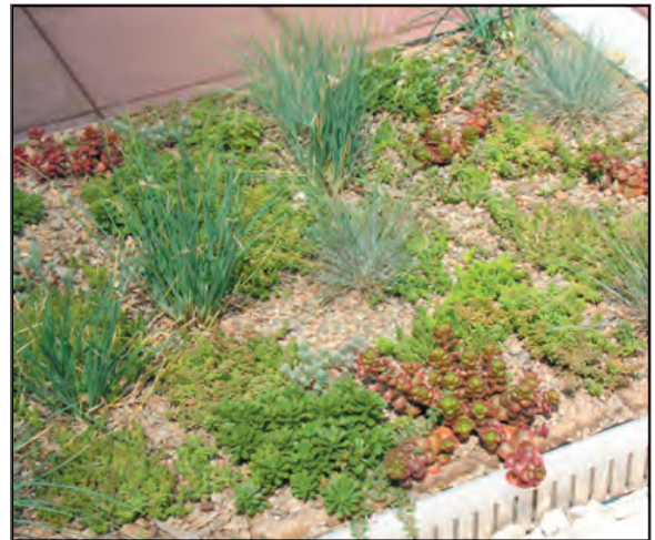
Figure 2-38. Example of plant types used in extensive green roofs. Photo courtesy of National Center of Excellence, Arizona State University.
