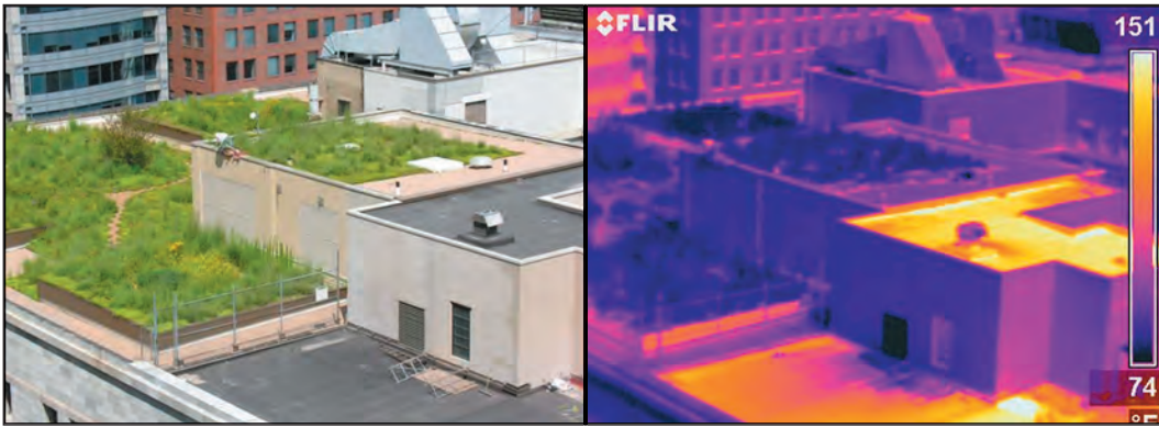
Figure 2-39. An intensive green roof on Chicago's City Hall. The infrared image on the right shows the dramatic temperature difference between a normal built-up roof and a green roof under identical conditions. The air temperature was around 85oF. Photos courtesy of National Center of Excellence at Arizona State University and Department of the Environment, City of Chicago
