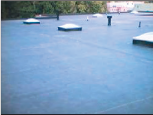
Figure 2-19. A fully adhered EPDM roof surface. Source: Kozlowski Co. ( http://www.kozlowskico.com/ )
