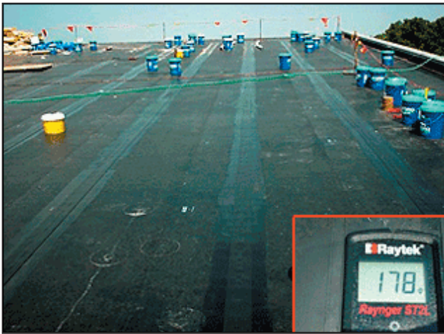
Figure 2-30. Cool roofing on a commercial low sloped roof. The surface temperature was reduced by 85°F after the roof was treated with a liquid applied cool roofing product. Images courtesy of Hydro-Stop, Inc.
