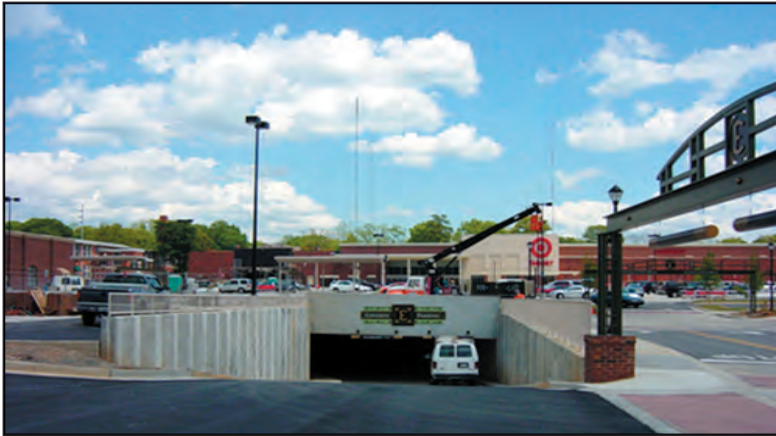
Figure 2-53. Example of underground parking in a commercial shopping center. Photo courtesy of Tunnerl-Spangler-Walsh & Associates.
