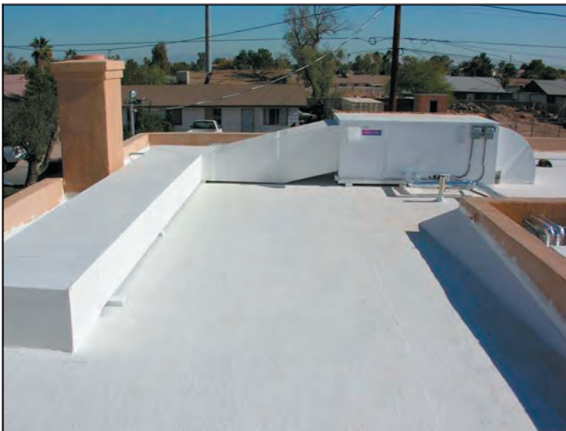
Figure 2-30. Cool roofing on a commercial low sloped roof. The surface temperature was reduced by 85°F after the roof was treated with a liquid applied cool roofing product. Images courtesy of Hydro-Stop, Inc.
