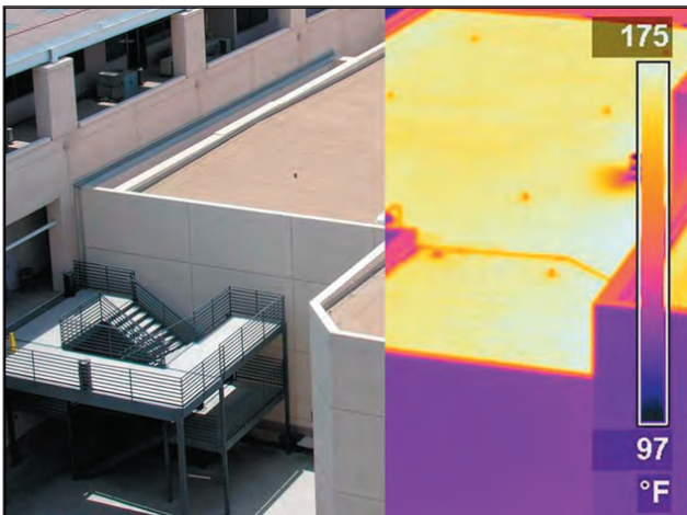
Figure 2-21. Modified bitumen on commercial, low-slope buildings. Photos courtesy of National Center of Excellence, Arizona State University.
