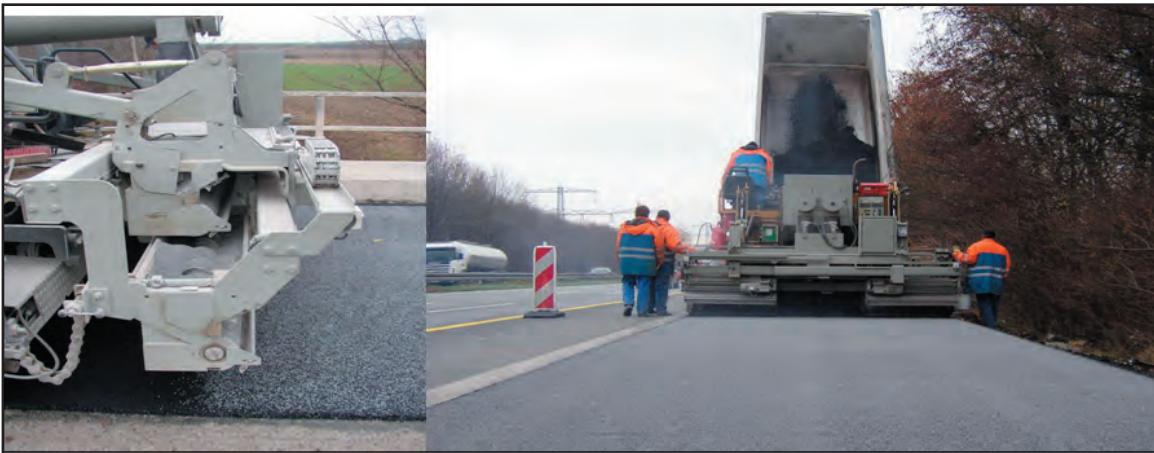
Figure 2-64. Gritting requires a spreading truck to deposit reflective aggregate to hot asphalt emulsion.
