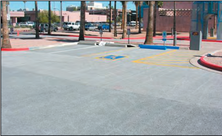
Figure 2-70. Pervious concrete parking lot outside of the Nelson Fine Arts Center at Arizona State University. Photo courtesy of National Center of Excellence, Arizona State University.
